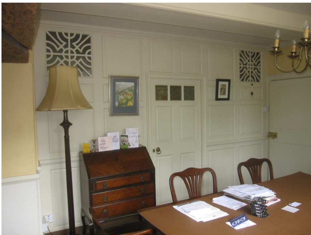
The panelled partition in the hall, with fretwork openings
