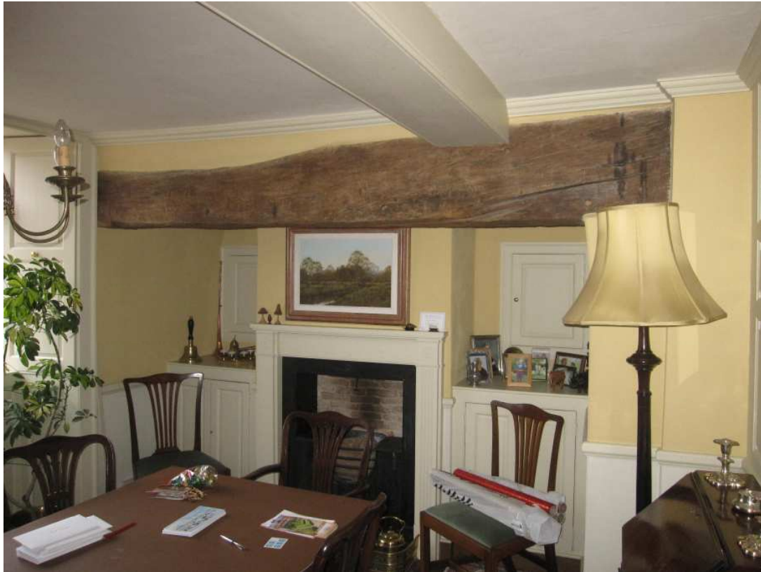
Inglennook fireplace in the north room (hall), with burn marks to right end of beam
