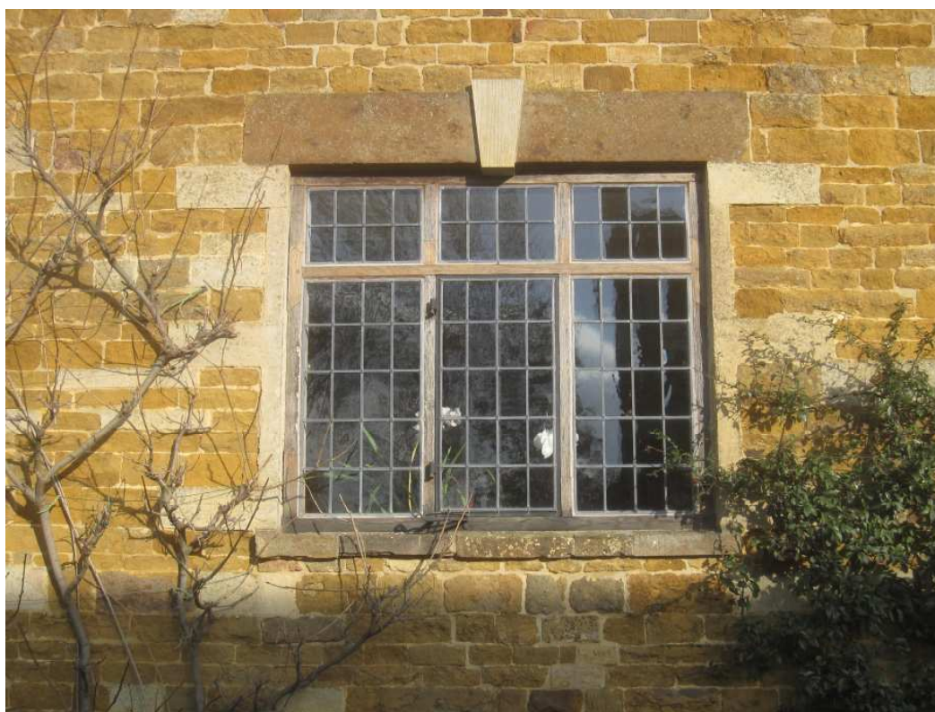
One of the original oak windows to the front elevation
