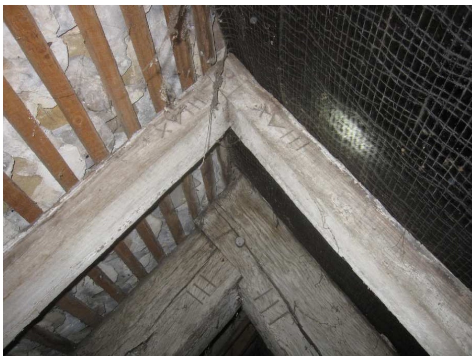
Carpenter's marks to the apex of truss T4 and adjoining rafter couple
